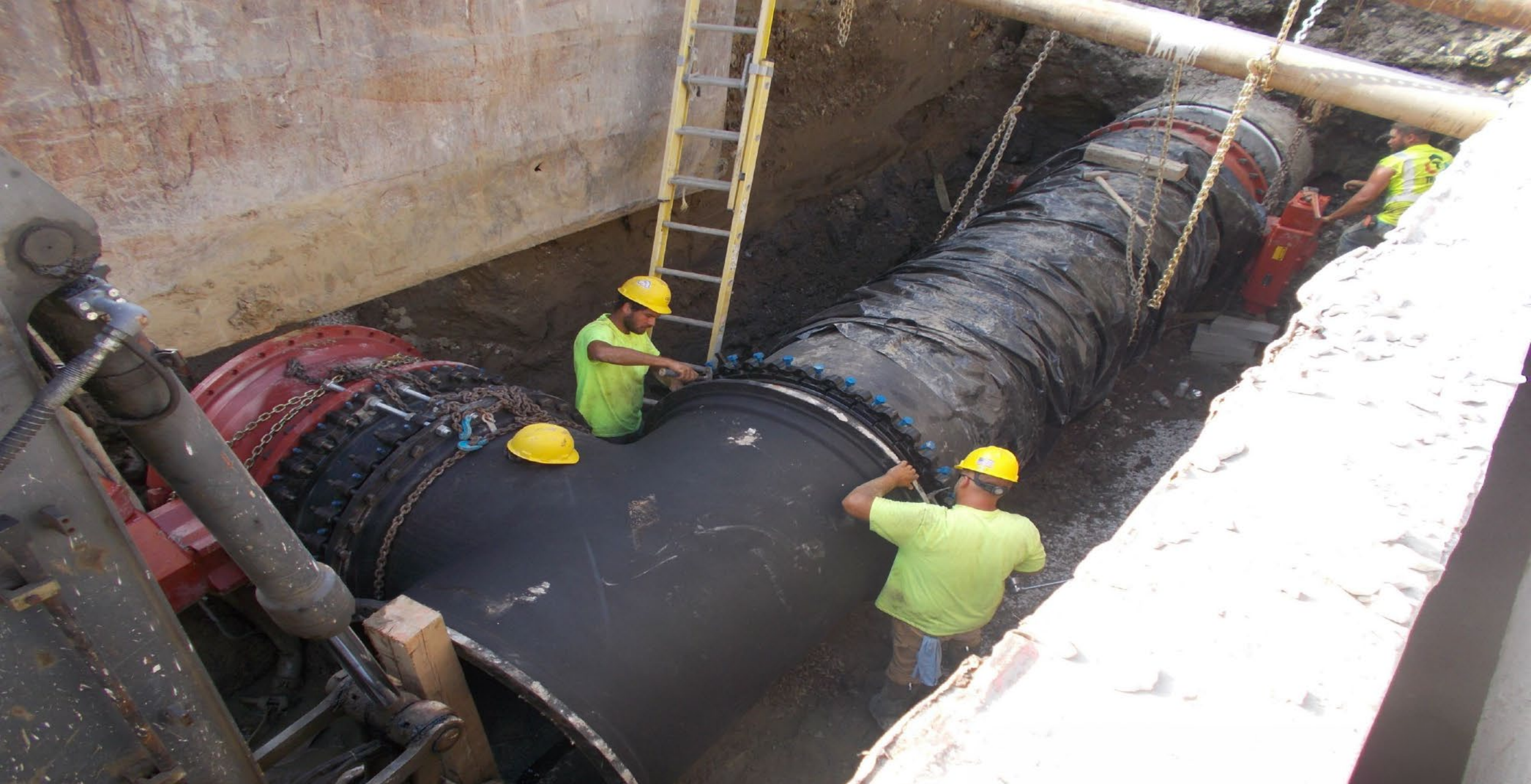
Pipe fitting installation
