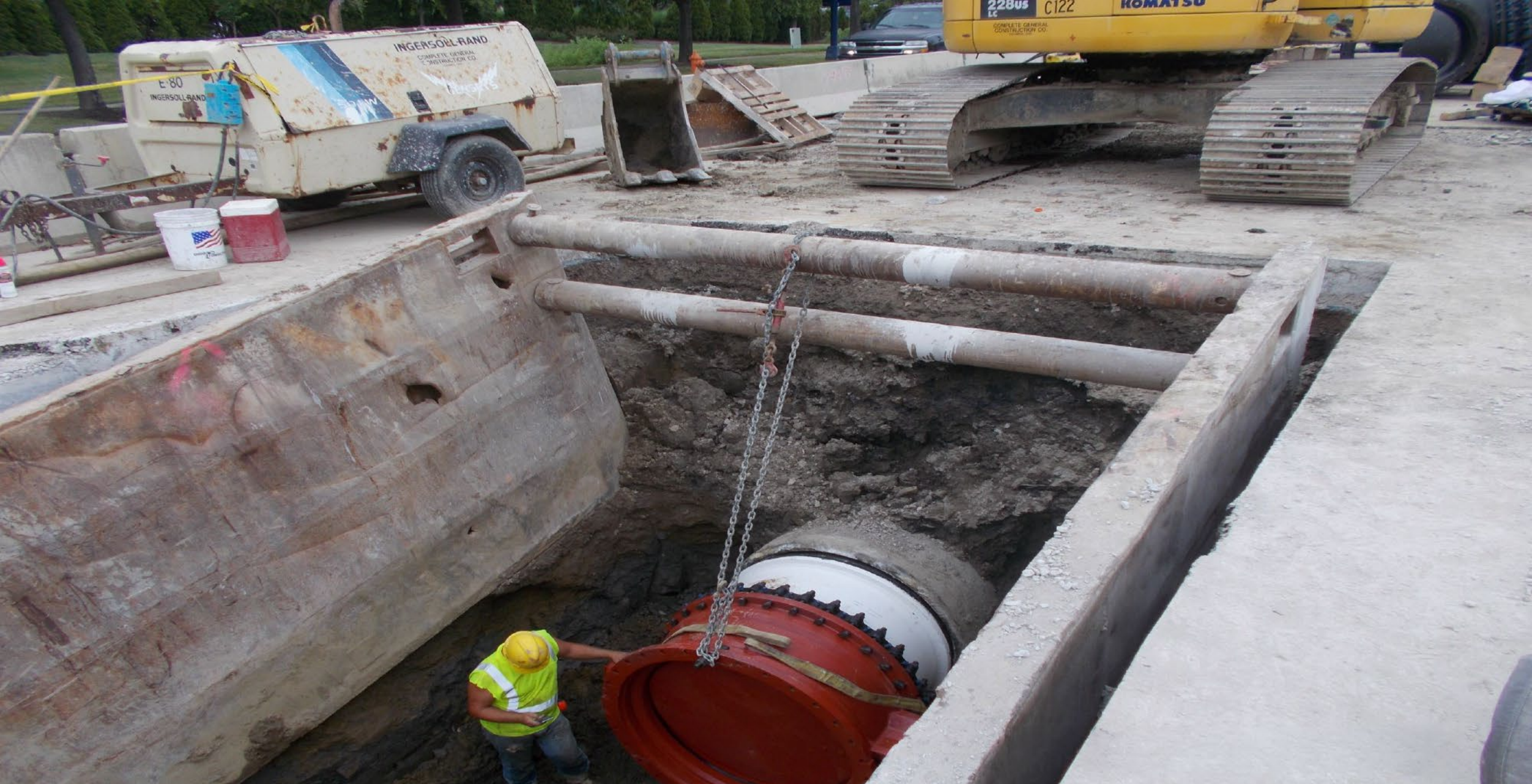
This is "open trench" construction
