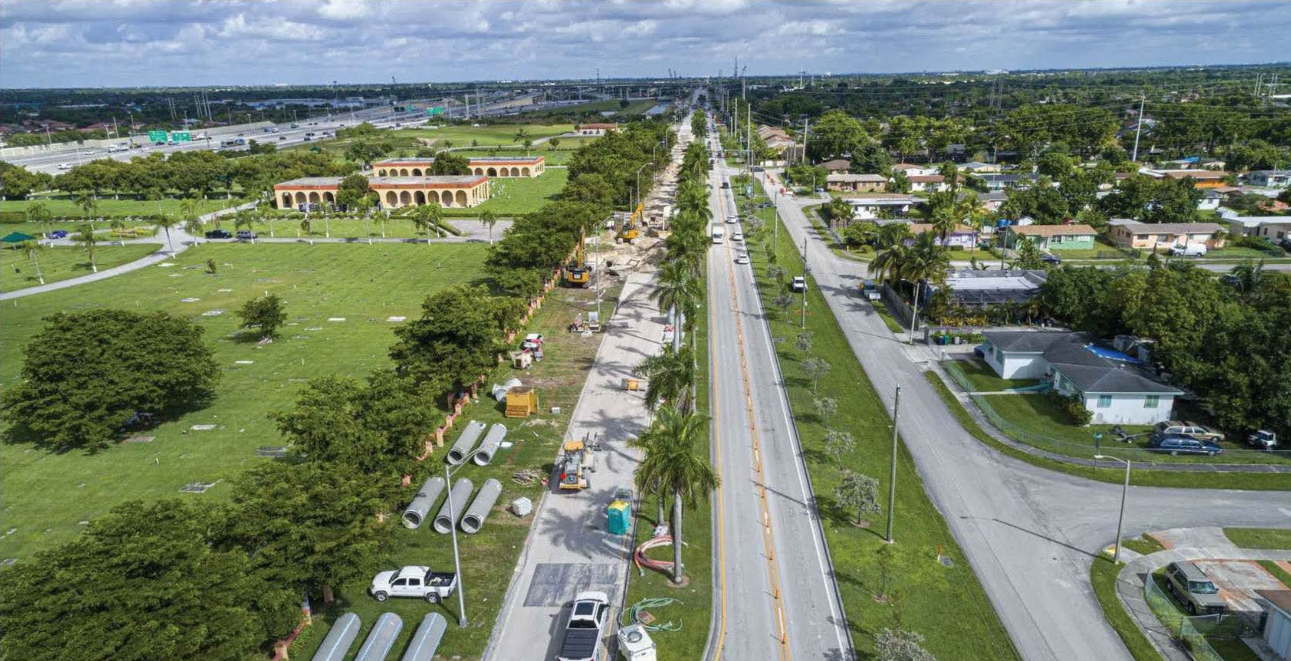
Example of space needs for construction and staging (Miami, FL)
